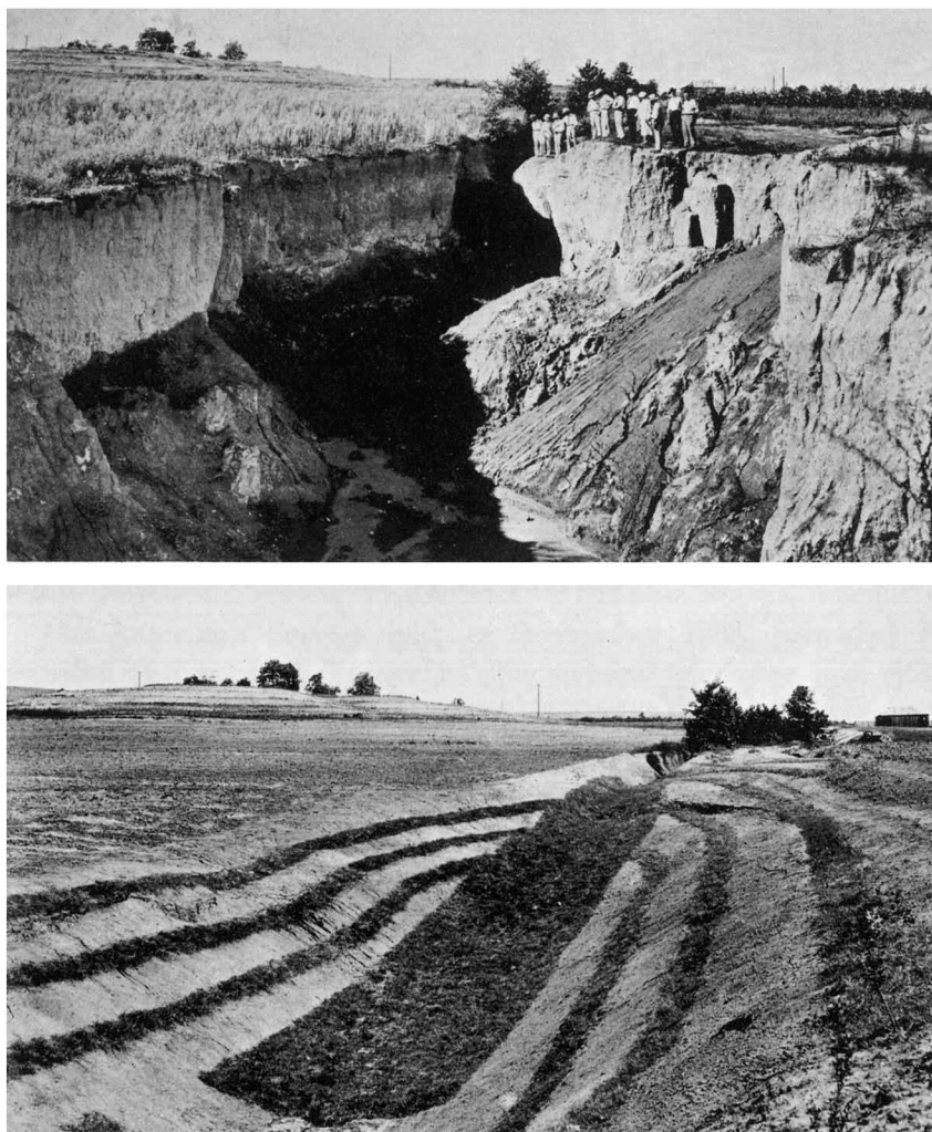
Fig. 18. A medium-sized gully on the South Tyger River Project (pm 5–7) in northwest South Carolina before and after the treatment in 1934 (Wilkerson et al., 1972, p. 18).
