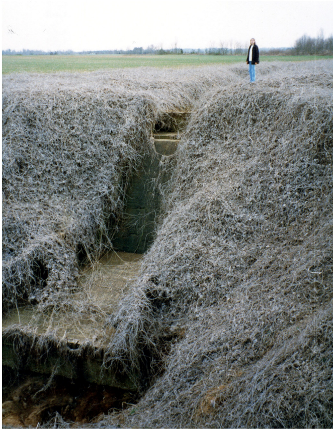
Fig. 19. A gully plug was set in concrete by the Civil Conservation Corps, probably in the 1930s, to prevent further gully head retreat (northern Mississippi, pm 5–8). Since then, the gully has deepened and widened. Today water slowly undercuts the plug and head retreat may occur again. The surrounding area is covered with Kudzu (picture taken on 15.02.1999 by the author).
