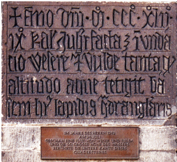
Fig. 3. Memorial stone at the St. Blasien church in Hannoversch Münden (pm 2–4) which documents the largest flood in central Europe between July nineteenth and 21st, 1342 CE. Translation: In the year of the Lord 1342, on the 24th July, a flood occurred on the Weser and Fulda Rivers, and the great height of the water touched the lower rim of this ashlar stone (picture taken on 15.07.2000 by the author).
