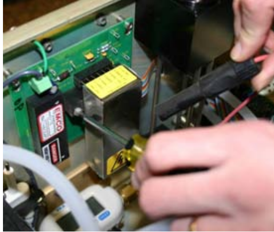
Figure 6-13 Removing High-Voltage Controller
