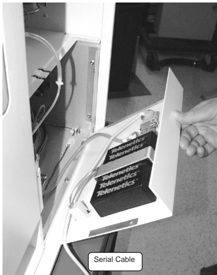
Figure J-4. Installing the internal modem assembly.
